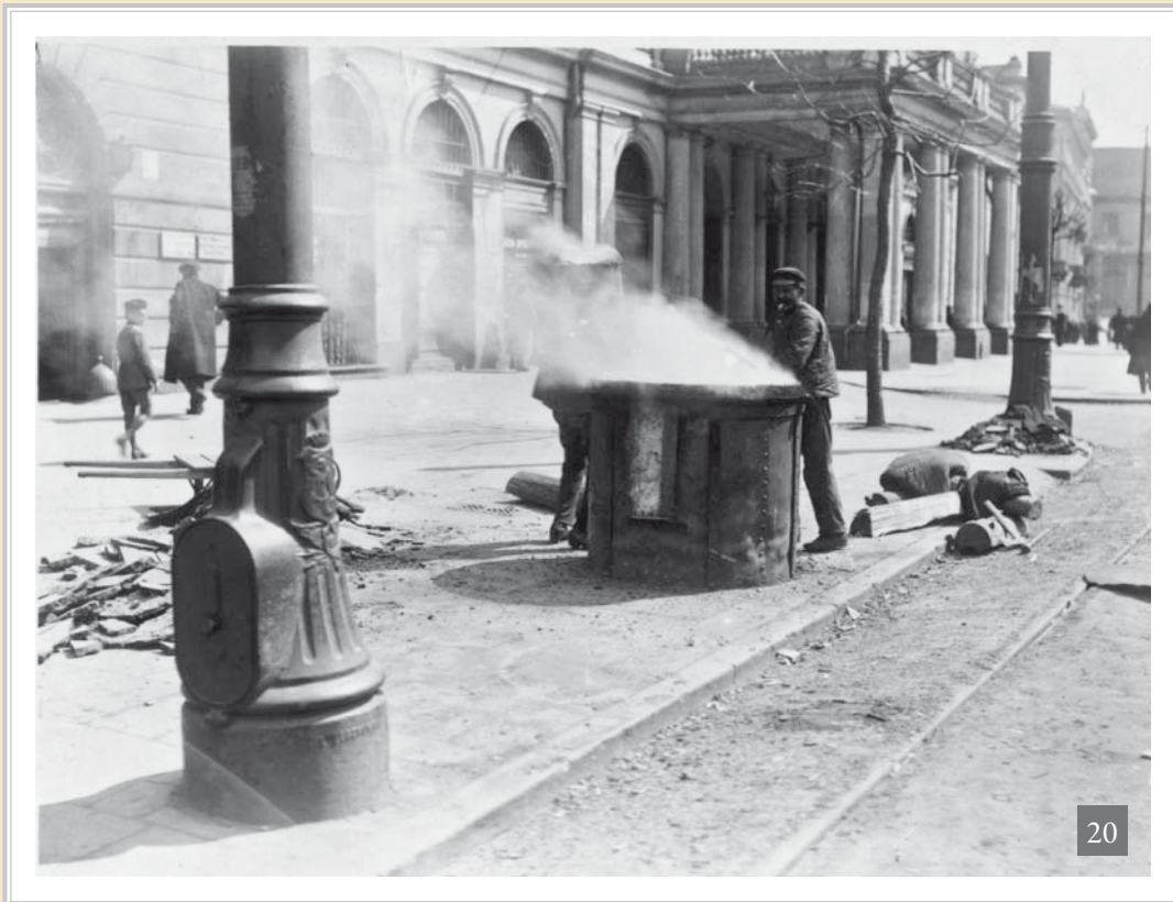
20 Remont nawierzchni przed gmachem Resursy Obywatelskiej (obecnie Dom Polonii), b.d. Renovation of the pavement in front of the Resursa (Citizen's Club, presently the Polonia Expatriate Center), not dated.
